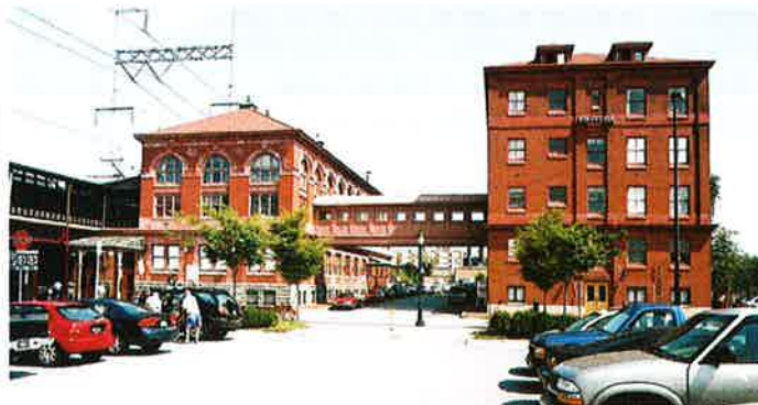
Wilmington Station connected to the Pennsylvania Office Building by a wrought iron bridge, which allowed PRR employees access to trains directly from their offices. It was dismantled in 2002. (James Tevebaugh photo)
